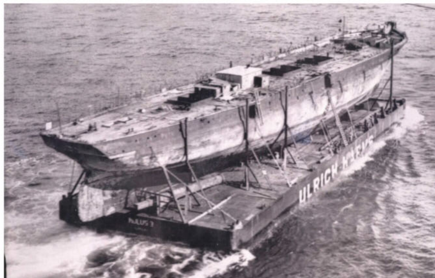
BELOW The ss Great Britain before restoration, being towed across the sea on a giant pontoon
