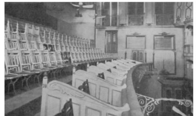
RIGHT In the refurbishment, the fans on the ceiling above the theatre were replaced with modern-day air conditioning
